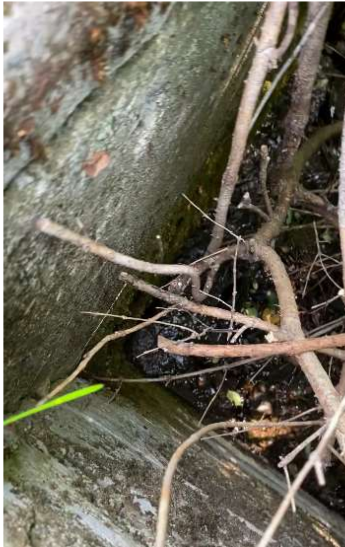
Near intersection of right concrete wall with right spillway training wall.
