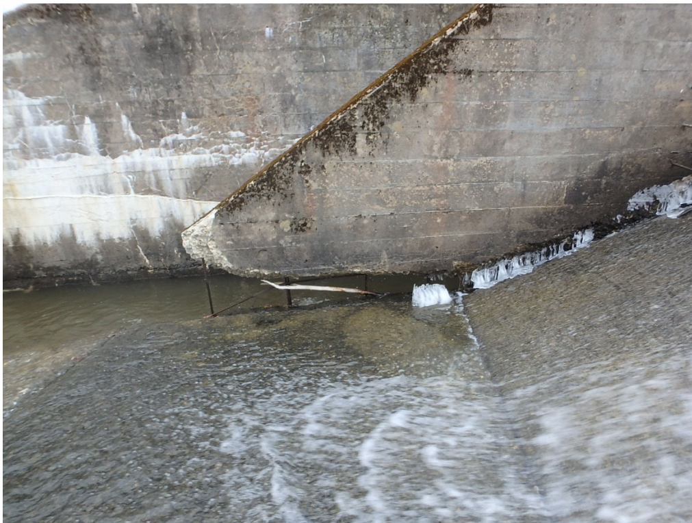
Photo 6: March 2021, downstream end of concrete wall separating the spillway from the outlet works, note continued section loss and deterioration.
