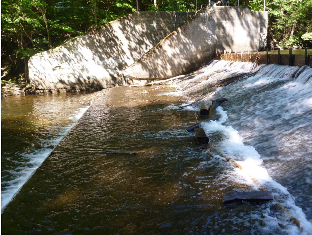
Photo 5: July 2019, downstream end of concrete wall separating the spillway from the outlet works, note continued section loss and deterioration.
