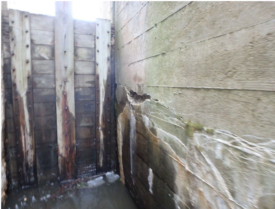
Photo 8: March 2021 looking upstream at the gate structure and wall separating the outlet from the spillway. Note the continued deterioration of concrete and displacement of the wall towards the spillway above the crack.
