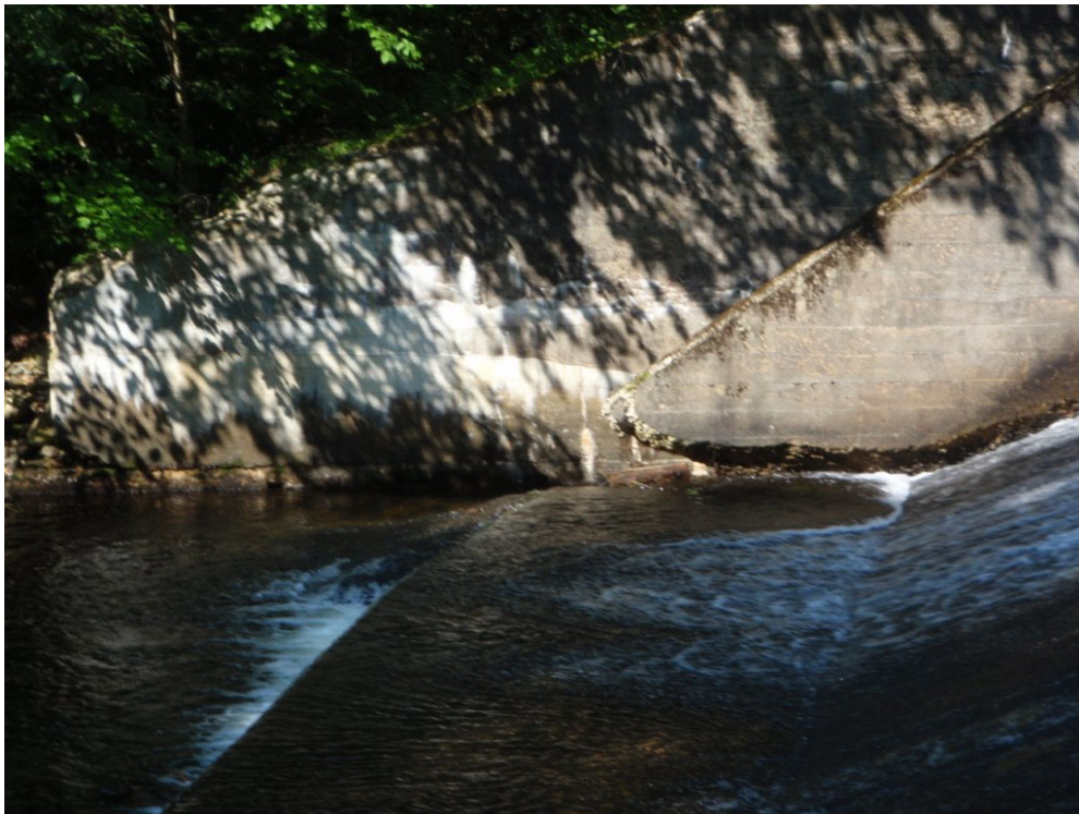
Photo 4: July 2014, downstream end of concrete wall separating the spillway from the outlet works, note continued section loss and deterioration.
