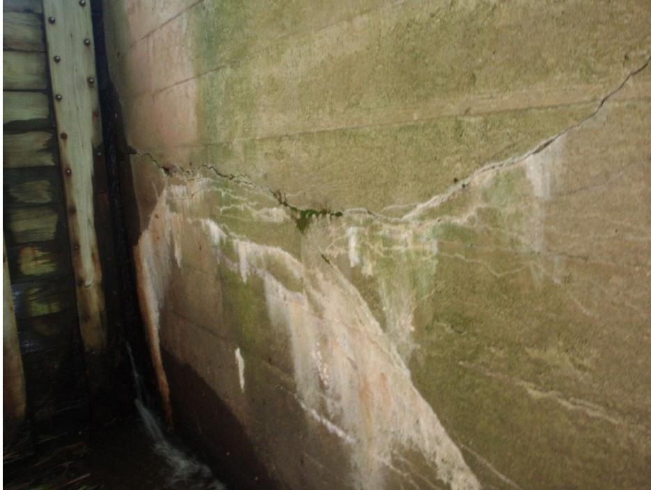
Photo 7: July 2014 looking upstream at the gate structure and wall separating the outlet from the spillway. Note the crack and deteriorated concrete.
