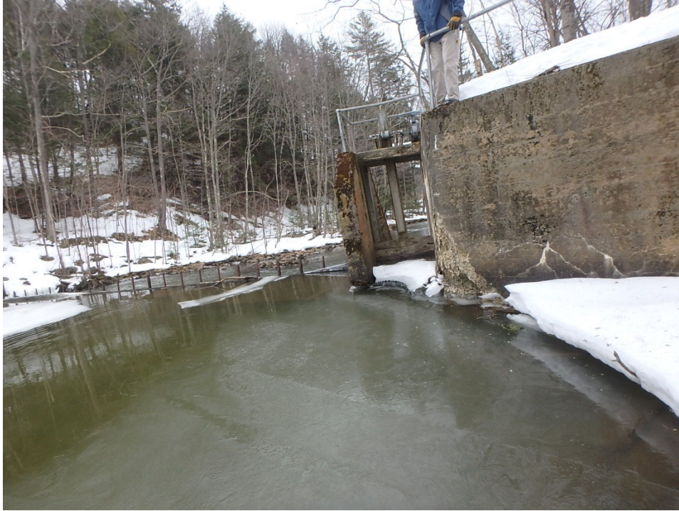
Photo 9: March 2021 looking downstream from the right abutment area. Note the section loss of the right training wall.
