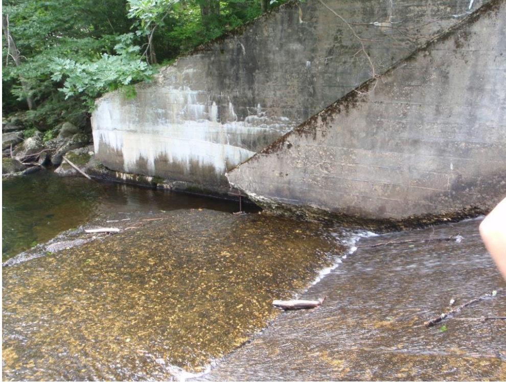
Photo 3: August 2010, downstream end of concrete wall separating the spillway from the outlet works.
