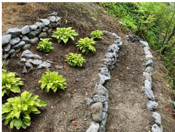
Installation of terraced gardens on a bank to filter and infiltrate stormwater.
