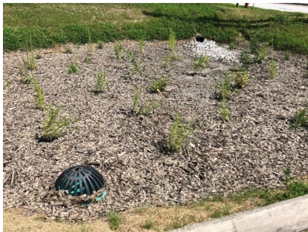
Bioretention structure installed to capture, treat, and infiltrate stormwater in Pittsford, VT.
