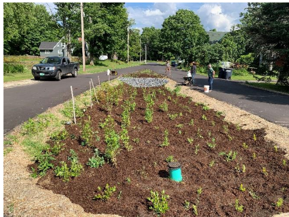
Bioretention structure installed on Prospect Street in Hyde Park, VT.
