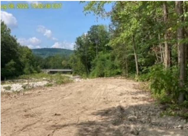
After berm removal, the river has space to move beyond its banks, allowing for natural channel evolution and reduction in erosive channelization.
