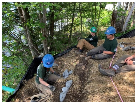
Installation of terraced gardens on a bank to filter and infiltrate stormwater.
