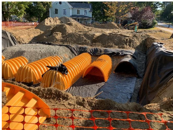
Subsurface infiltration system being installed at Copley Park in Morristown, VT.
