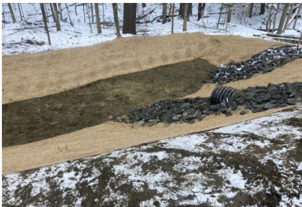
Infiltration trench installed along the roadside at Hubbard Park in Montpelier, VT.
