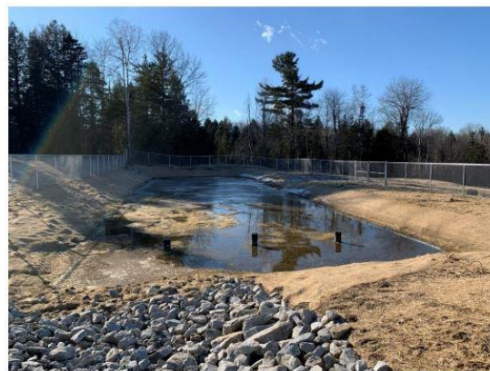
Stormwater infiltration basin constructed at the Barre Town Recreation Fields in Barre, VT.
