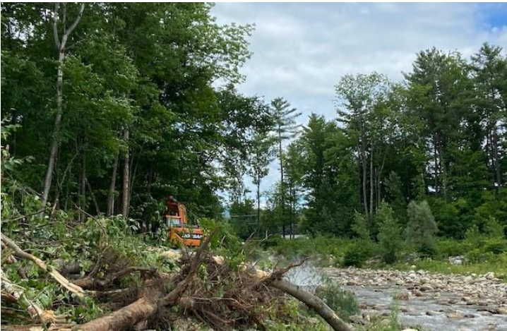
A berm along side the Cold River prevented the river from accessing its floodplain. Work underway to remove the berm.
