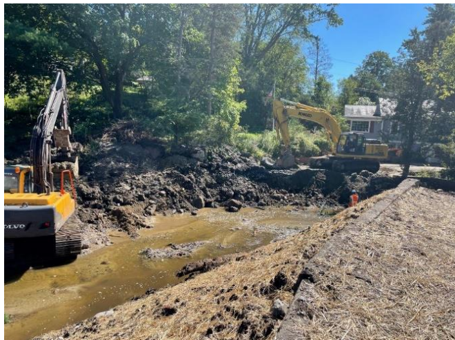
Removal of the 75 ft long and 10ft high stone rubble and concrete barrier dam on Tenney Brook.
