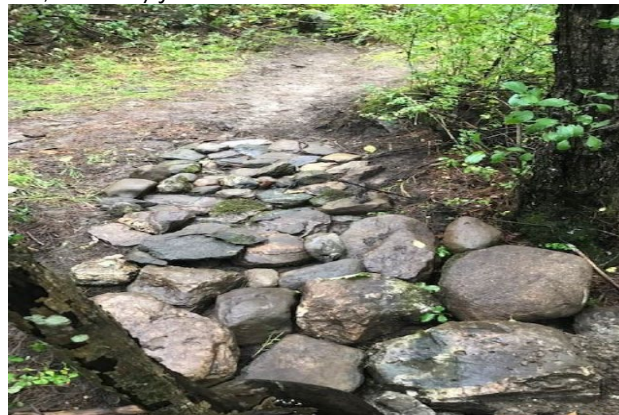
Eight drainage control structures were installed on this Class IV road in Hinesburg, VT. Structures help to stabilize eroded areas.
