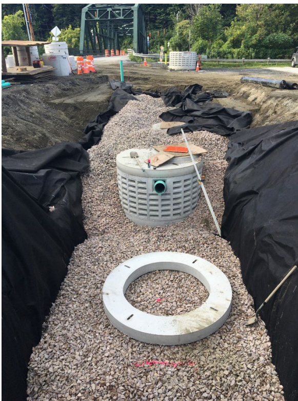
Installation of a dry well along Taylor Street will increase the city's capacity to retain and treat stormwater runoff.
