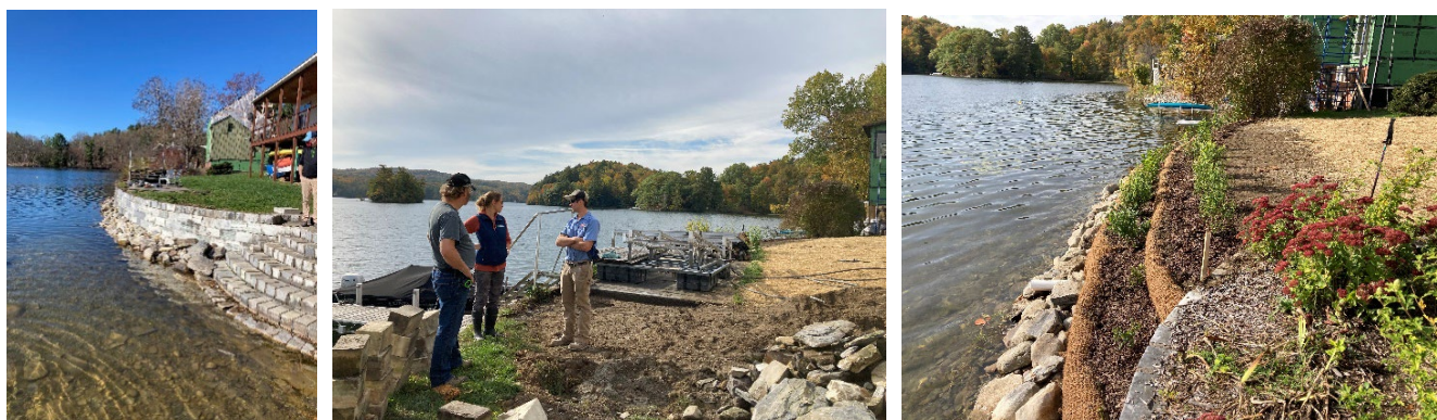
Figure 4. Before (left), during (center) and after (right) installation of a Lake Wise project showing fiber coir roll toe placement with an erosion control blanket along Lake Hortonia in Sudbury, VT.
