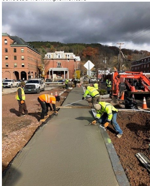
After the installation of drywells and rain gardens, crews are re-installing the sidewalks along Taylor Street.
